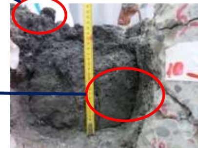
After Removing Majority of Molten Substances
